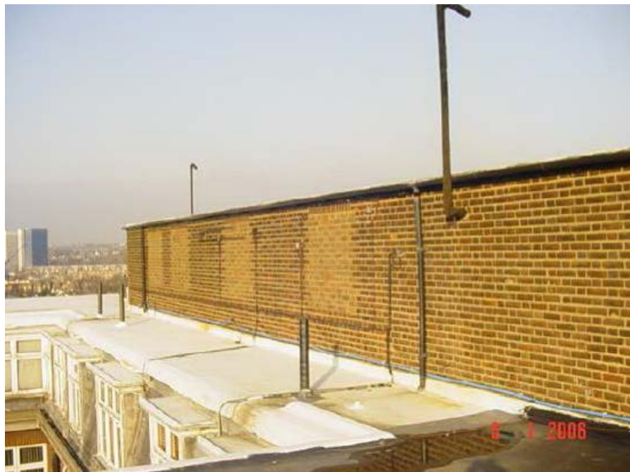
View of front (south east) and side (south west) elevations (top) and view of bricked up fenestration to south western elevation to be opened up (bottom).
