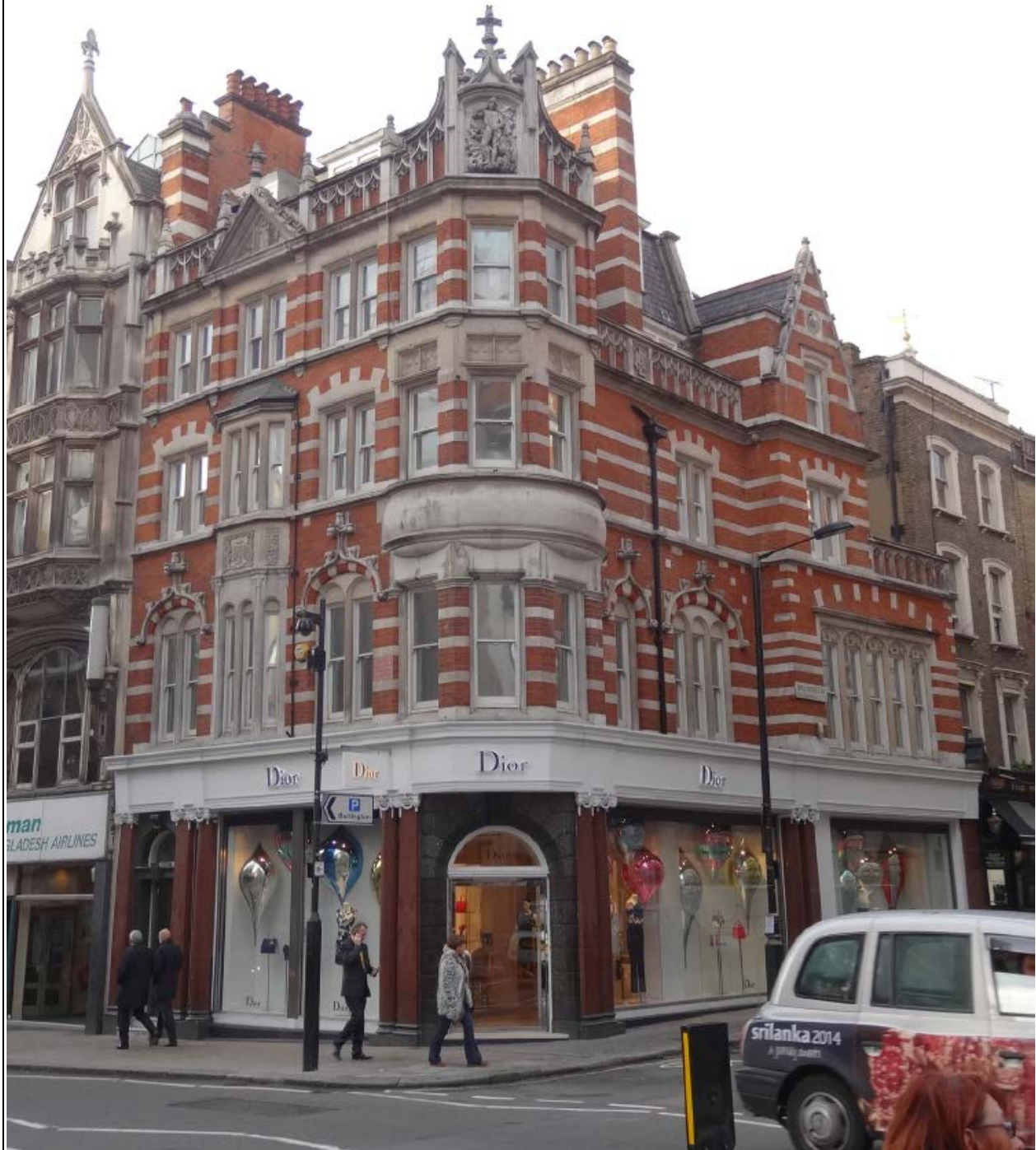
Photograph 1. View of Conduit Street and Mill Street frontage showing proposed grilles
